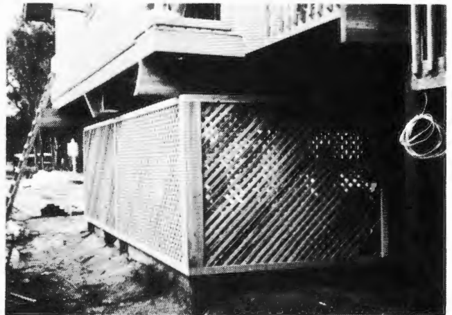
Figure 4.54. Breakaway Walls
